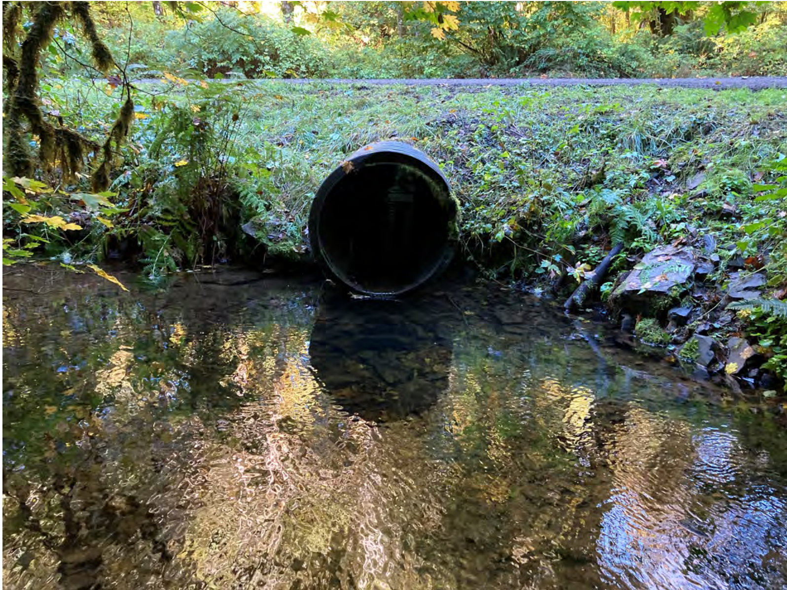
Swartz Creek Unnamed Tributary: downstream of culvert 10/18/2023
