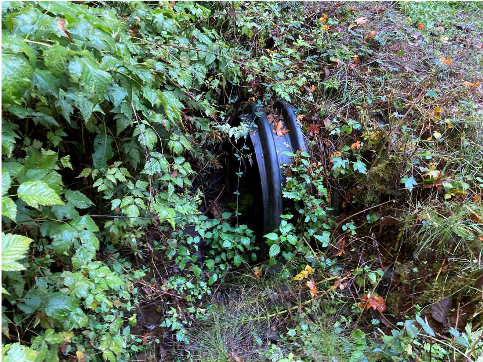
Swartz Creek Unnamed Tributary: upstream of culvert 10/18/2023
