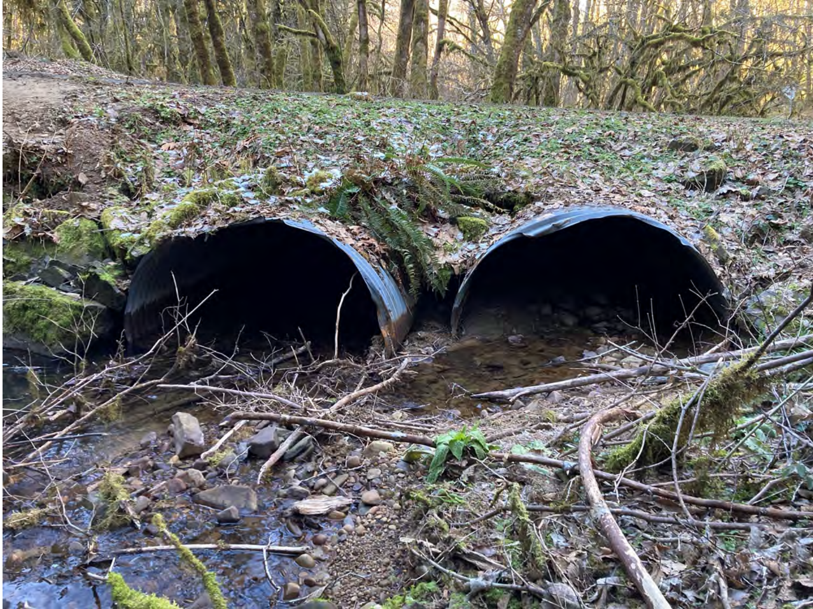
Swartz Creek mainstem: upstream of culvert 2/23/2023
